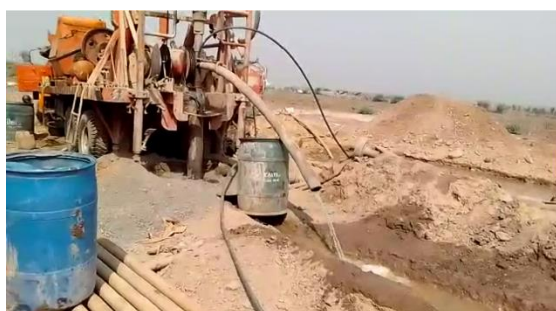
Figure-5.55: Development of Tube Well for Mr. Gul Said Tube Well & Solarization of Tube Well in Maraje Mankisharif, Nowshera
